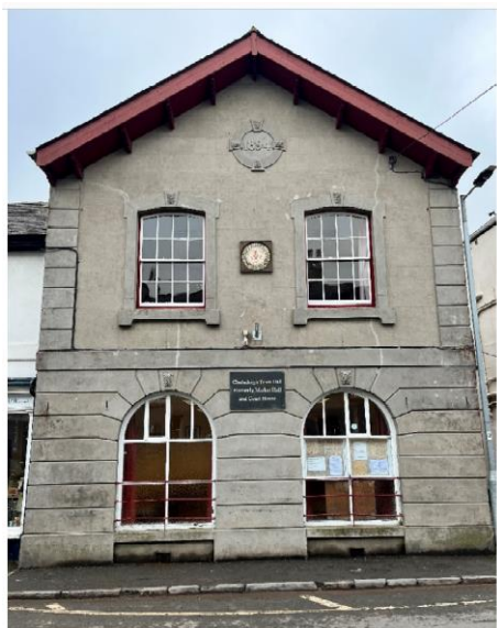
Exterior of building
