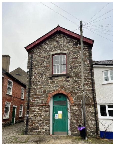
Exterior of building
